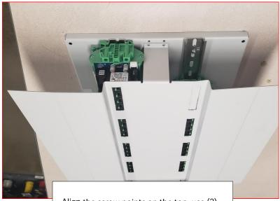
Align the screw points on the top, use (2) sheet metal screws to secure the dead front cover tab to the backplate.
