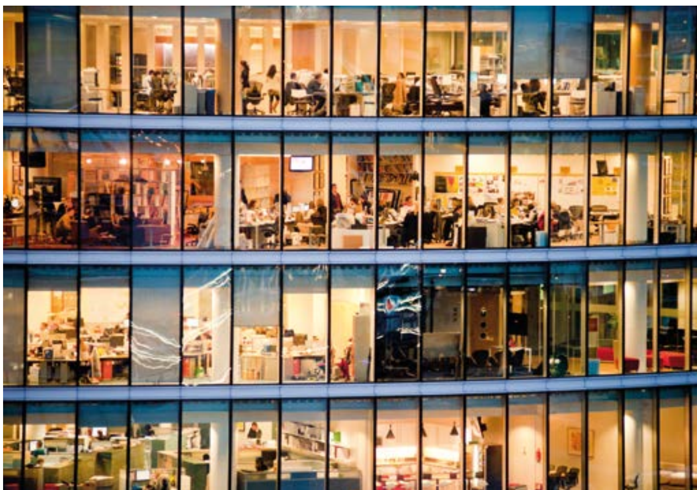
Occupant centric controls for the modern commercial office space
