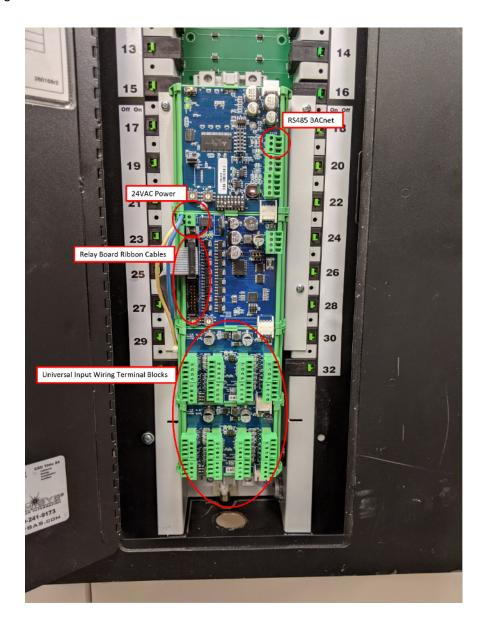
5) After all wiring is verified, energize the circuit breaker feeding the 24VAC transformer and begin configuring the CM control module for lighting sequencing and operation.
