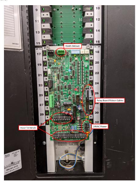
2) To remove the controller board, loosen the two thumb screws above the board as shown and pivot the mounting plate out from the panel.
